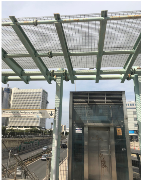
Figure 3. Elevator and stairs leading to the station
