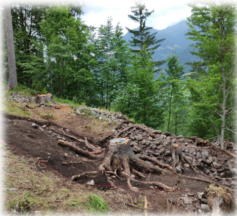
Part of the excavation
